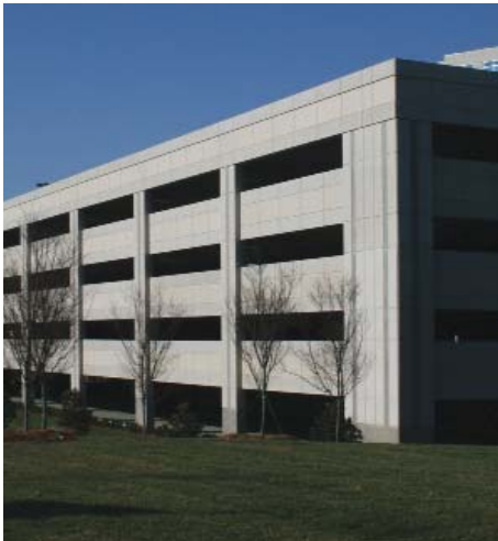
Ballantyne Garage Charlotte, N.C. Precaster: Metromont Corporation
