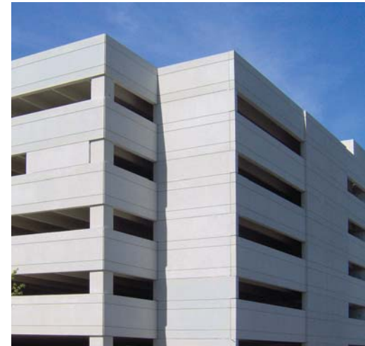
Children's Place Garage Secaucus, N.J. Precaster: High Concrete Group LLC
