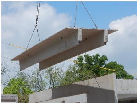
The podium deck typically acts as both a structural floor and as a transfer slab for the framed construction above. Precast used in multi-family projects provides inherently high fire ratings, with reduced vibration and sound transmission.
