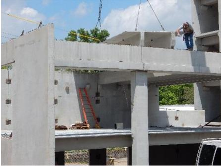
Whistlebury's residential complex features multiple stories of wood frame construction over an elevated concrete parking deck. The podium design provides a cost-effective solution with design flexibility, speed of construction, and reduced environmental impact.
