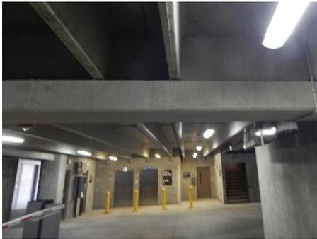
Interior framing utilizes double tee, beam, column, and shear wall construction. The load-bearing architectural precast envelope consists of buff-colored sandblasted concrete panels.
