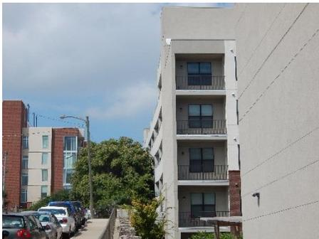
An architectural concrete mix of local aggregates and sands was given a sandblasted finish to ensure that the color and texture of the new addition would match those of the anchored apartment building and retail shops. Sandblasting is an economical solution for creating blended and uniform color in precast panels. This unique solution reduces the need for additional coatings, while providing a nearly maintenance free exterior.
