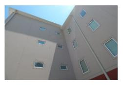
Flat insulated wall panels frame the outside of the building. The wall panels are designed for thermal efficiency to stabilize interior building temperatures. The panels on floors two through four are sandblasted and then painted to match the buildings throughout the campus.
