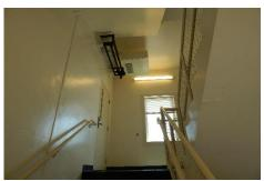
Precast stair components are featured in the dormitory project. The standard gray walls are painted to match the interior drywall and framing. The stair boxes have openings placed at each entrance of the different floors.
