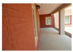
A brick printed form liner is used to create a ground level outcropping. The precast is then painted to match existing campus structures. The multi-textural finish allows the precast structure to function both structurally and aesthetically.
