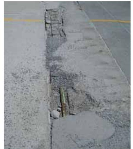
Cast-in-place garages are susceptible to deck corrosion, which can lead to durability issues and water infiltration.
