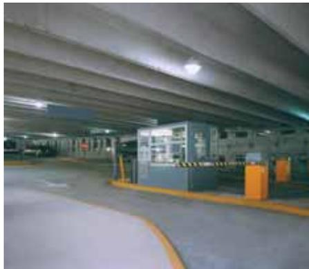
The use of C-GRID in the double tee flange eliminates the need to use sealers or corrosion inhibitors.
