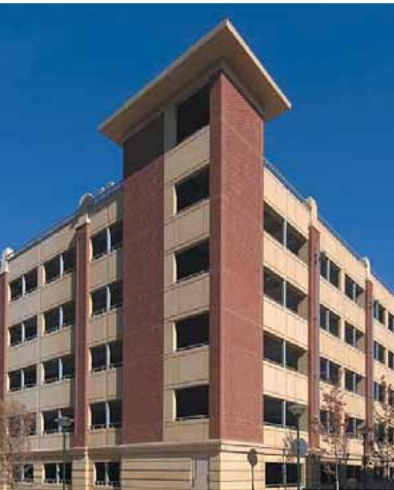
Delivered ready to erect, CarbonCast® Double Tees avoid the costly scheduling, quality and safety issues associated with coordinating the many trades required to complete a cast-in-place deck. They also minimize weather delays and site congestion caused by laborers and stored materials and equipment.
