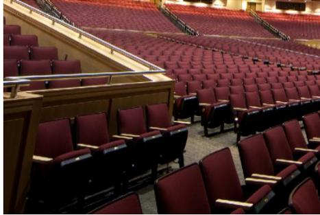
The auditorium's precast prestressed risers are built in single and double riser sections on steel raker beams and house seating for 15,000 attendees.
