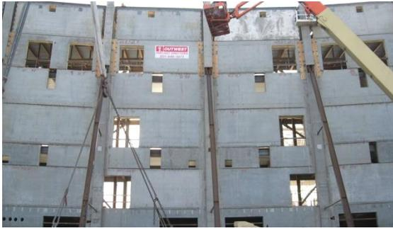
The walls were cast in a vertical battery mold to prevent movement of the voids and give form finish to both sides. Casting integral openings into the panels allowed for a single-unit design to reduce the number of pieces needed. Fewer walls decreased casting and crane time for a more efficient structure.
