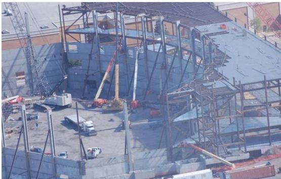
Once the columns were erected and braced, installation of the 16" thick precast voided wall system began. These unique wall pieces contained voids to reduce their weight, allowing larger pieces to be shipped and erected. For a scale of reference, the back wall was set at a 266'-3" radius.
