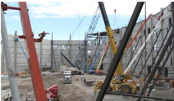
The conversion from cast-in-place to precast saved both construction time and costs. The cast-in-place design may have required an onsite concrete plant due to the project location and the availability of concrete. Utilizing a precast solution, the owner saved what could have been a large expense for this plant mobilization.
