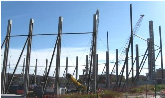
An extensive bracing system was designed to support the wall until the wet joints were completed and reached the required strength. Cables were used to restrain all in-plane forces on the wall during construction.
