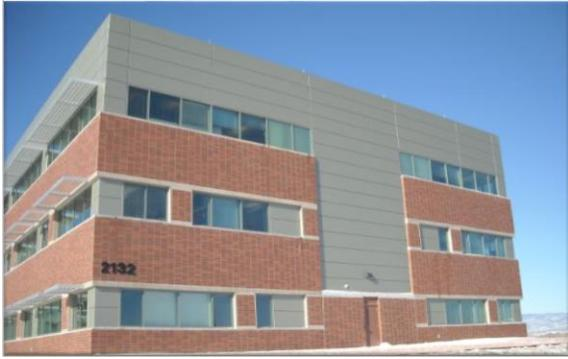
The exteriors are clad with integral thin brick in a three color blend. The aesthetic thin brick is designed to incorporate the structure into the existing Fort Carson architectural landscape.
