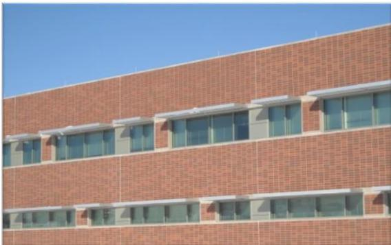
The headquarters building features a significant number of windows that are also blast resistant, with the anchoring to the precast spandrels designed to take significant blast loads.
