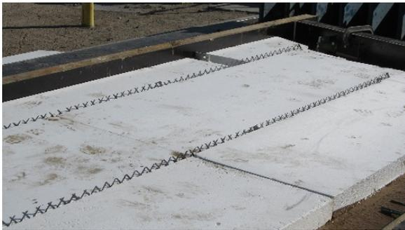
CarbonCast® architectural panels can be designed with infill insulation to reduce the weight of the enclosure system, as well as provide thermal efficiency and concrete mass on the interior of the structure.
