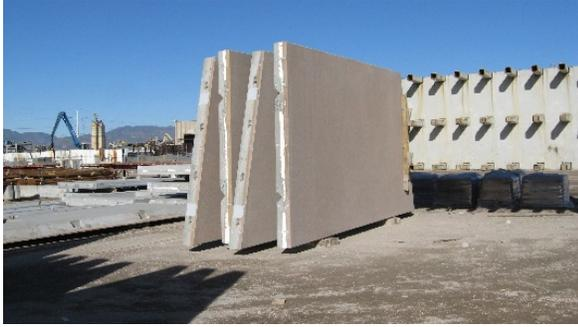
EnCon Utah created insulated high performance precast shear walls with CarbonCast® C-grid® to meet Clark County's thermal efficiency requirements.
