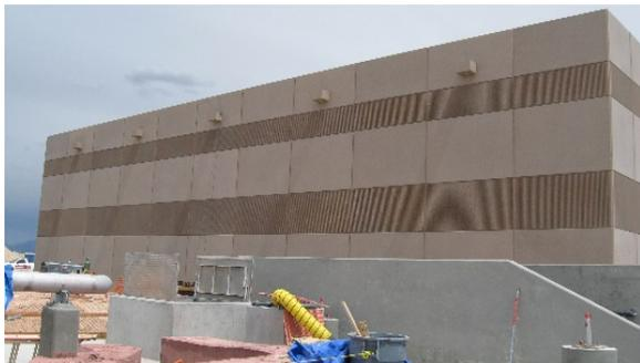
Epoxy rebar reinforcement and stainless steel connections were used for panel installation.
