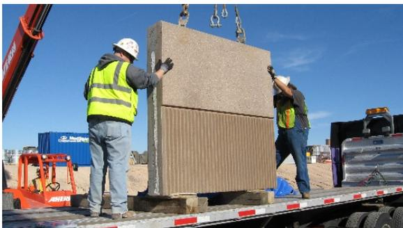
CarbonCast® architectural panels are designed with edge to edge insulation to provide a complete thermal building wrap with no cold zones or thermal bridges.
