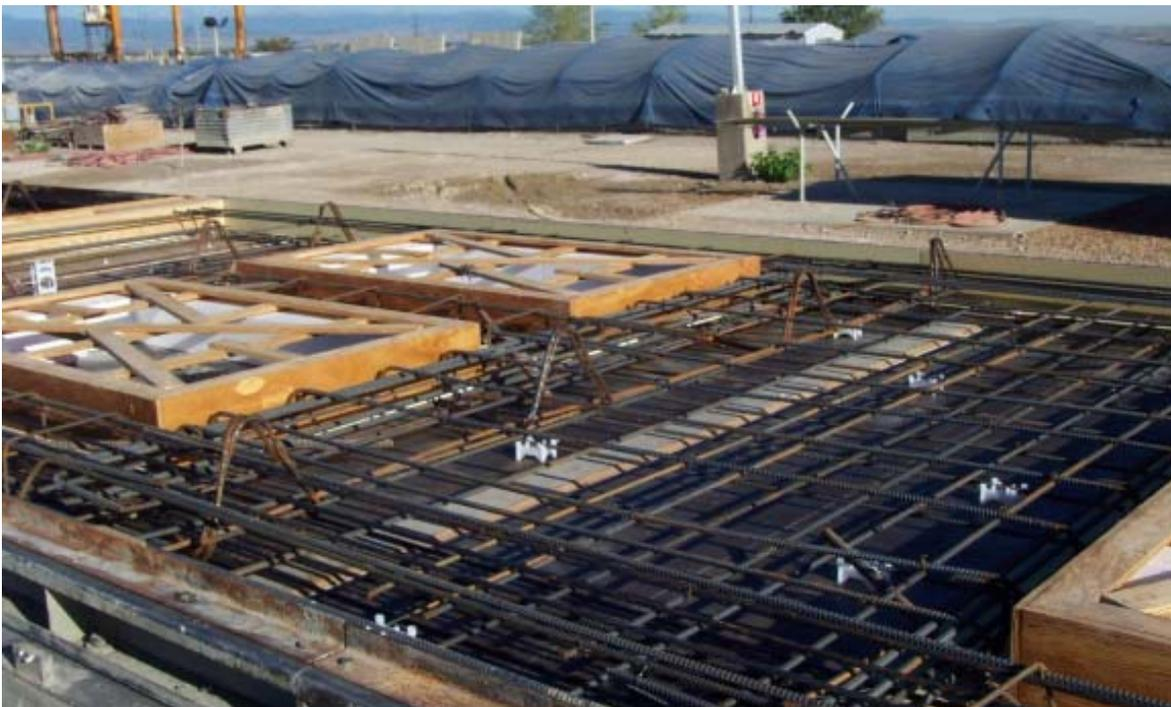
100% of the forming and reinforcement is complete. Awaiting inspection and casting.
