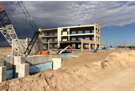
Using a tower method to erect the 168,000 square foot facility, the entire height of a bay is erected before moving to a new bay. This permits faster turnover to the general contractor, which allows site work of other trades to begin long before other construction methods could provide.
