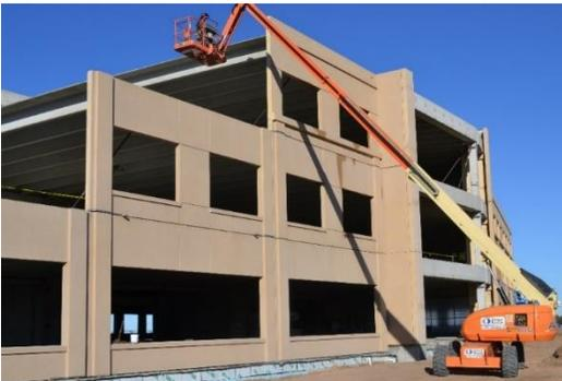
An exterior elevation during erection shows precast panels functioning as the load bearing structural elements. Precast concrete enclosure walls are an integral part of the envelope design and integrate moisture, air and vapor barriers for added control, performance and functionality.
