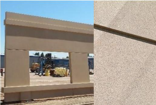
Panels are being processed for finishing with a light acid etch. This process involves removing the thin skin of cement matrix from the panel surface and exposing the fine architectural aggregate.
