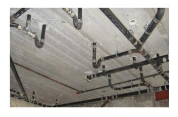
Large open spaces are created when using hollow-core. Spans of up to 40'-0" were achieved on this project over the cart barn storage. Pre-manufactured slabs enabled the contractor to have immediate access to the covered portion without the obstacle of shoring, common with other methods of construction.
