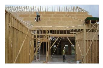
Framing was performed immediately after the topping slab was poured and cured. Line loads of the structure above were coordinated and camber monitored to ensure that the structural slab was performing as designed.
