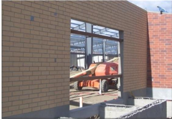
The high performance, thermally efficient, insulated wall panels are produced with CarbonCast® carbon fiber shear grid. The use of the carbon fiber wythe ties and insulation creates a wall system with no thermal breaks, thus providing a steady state R-value.
