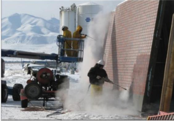
Plant fabrication allows panels to be manufactured even in the worst conditions. Casting, stripping, and field finishing are all performed at the casting facility. Wax is washed off the panels at the plant before transporting them to the job site.
