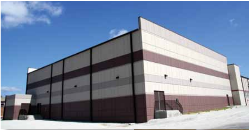
The Dallas County School District in Buffalo, Mo., created a FEMA safe room for students during construction that added onto its gymnasium.
