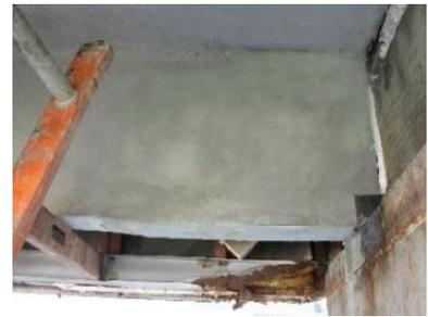
Forming pieces are installed to pour the new double tee stem with a high strength non-shrink grout. The new double tee leg is shown after pouring. The concrete area is then cleaned, patched, and finished.
