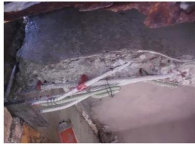
Before repair the concrete surface is prepared. This process includes removing damaged concrete and installing new steel reinforcement, and the application of corrosion inhibiting bonding agent.
