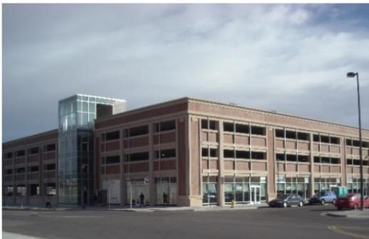
Architectural aluminum tubes continue the vertical lines established by the storefront mullions. Recesses were cast within the spandrel bull nose to facilitate the attachment of the tubes. Various textures, colors, materials, and finishes combine and contrast to create a building that is as appealing as it is functional.
