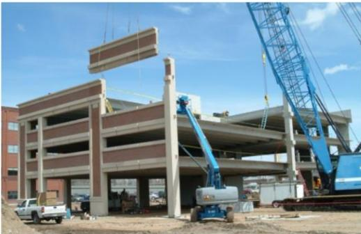
The interior framing utilizes double tee, beam, column, stair, and shear wall construction. The load-bearing architectural precast skin consists of buff-colored acid etched concrete and red-brown modular-size thin brick.
