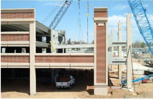
The exterior of the structure is supported by 42-foot long architectural precast columns, two feet deep by six feet wide. To achieve a continuous smooth surface, the massive columns were cast in one piece without splices.
