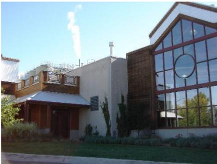
The sandblast finish on the precast wall panels it complements the rustic wood office building components and blends into the brewery's natural environment.
