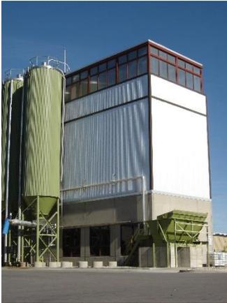
Industrial grade precast panels were selected and a sand blast finish was delivered on site after panel erection. The resulting finish is a light to medium blast, barely showing the aggregate.
