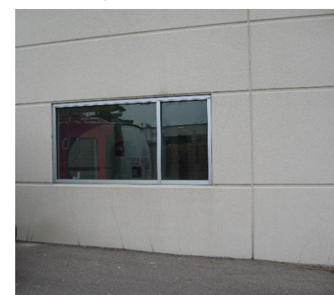
3. Window/door conversion - Before
