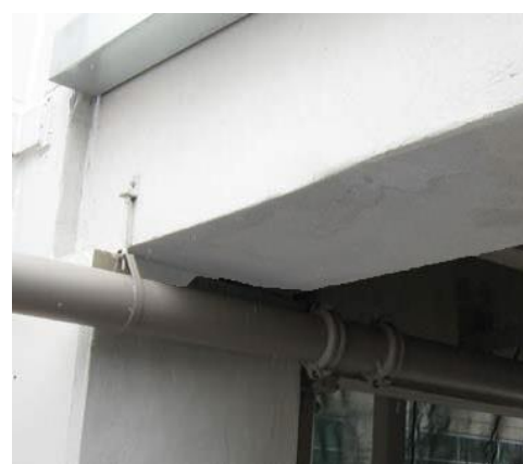
2. Parking structure beam - After
