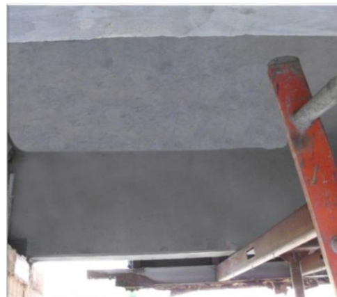
1. Double tee bridge repair - After
