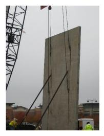
Tilt-up panels are cast and cured, and braces are installed prior to tilting panels into position.
