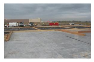
Field layout is the first step of the process to identify setup and position of panels prior to casting on the slab.
