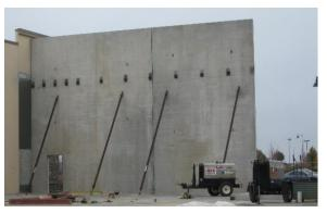
An advantage of tilt-up is that the joist beam seats are welded on the ground rather than the air, saving time and money.
