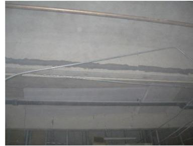
In order to change the double tee live load capacity from 75 psf to 125 psf to meet requirements, carbon fiber rods were integrated into the double tee legs.
