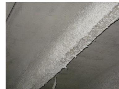
EnCon Renew used fireproofing finish on the double tees to provide the necessary two hour fire rating.
