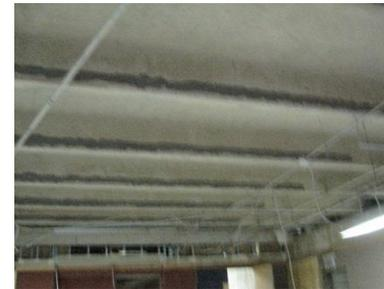
To install carbon fiber rods for reinforcing, grooves are saw cut into the concrete surface slightly larger than the diameter of the rod. Epoxy was used as a structural adhesive to bond the carbon to the concrete.
