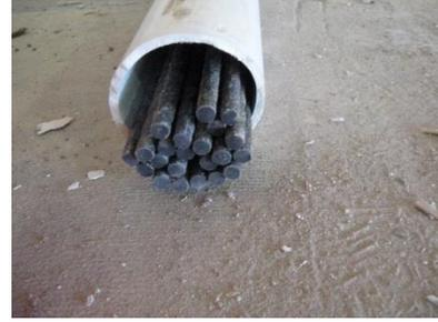
Carbon fiber rods were placed in the bottom leg sections of both sides on the double tee legs. The carbon fiber rods act as reinforcement to increase live load capacity.
