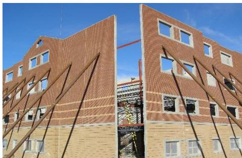
The structure's 18,249 square foot exteriors are clad with thin brick, split-face concrete masonry units with an architectural banding. The versatile precast wall panels provide lateral shear load resistance and adhere to a steel frame structure.
