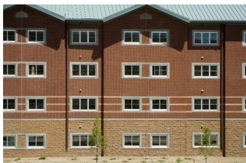
The wall panels are designed to house a significant number of windows to maximize daylight in the offices that line the perimeter of the buildings. Because the exterior walls are precast, the windows are simply anchored within the rough opening cast into each panel.
