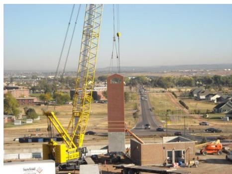
Precast concrete was used for this project because of significant time savings and labor costs. The panels were cast at a nearby plant, shipped to the project site, and quickly erected. The significance of this unit's mission, and the rapid pace of returning soldiers, required that new facilities be erected quickly to keep pace with the demand for services.
