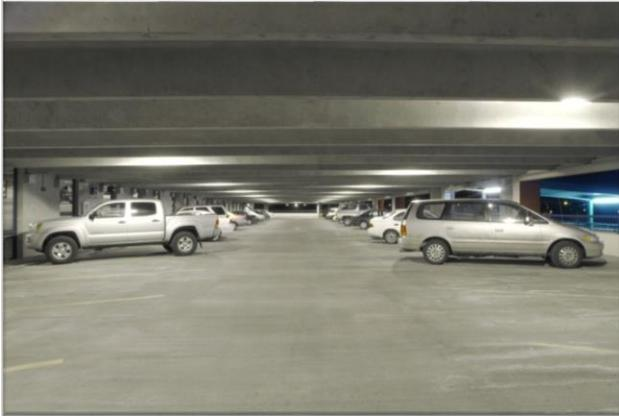
The parking garage consists of an architectural and structural precast concrete structure approximately 360 feet by 240 feet in design, with three supported levels providing 908 parking spaces. Design features include ornamental brick exterior elements and tower features to identify the structure with two glass back elevators. The building is user-friendly and completely accessible to meet the transportation needs of the disabled community.
