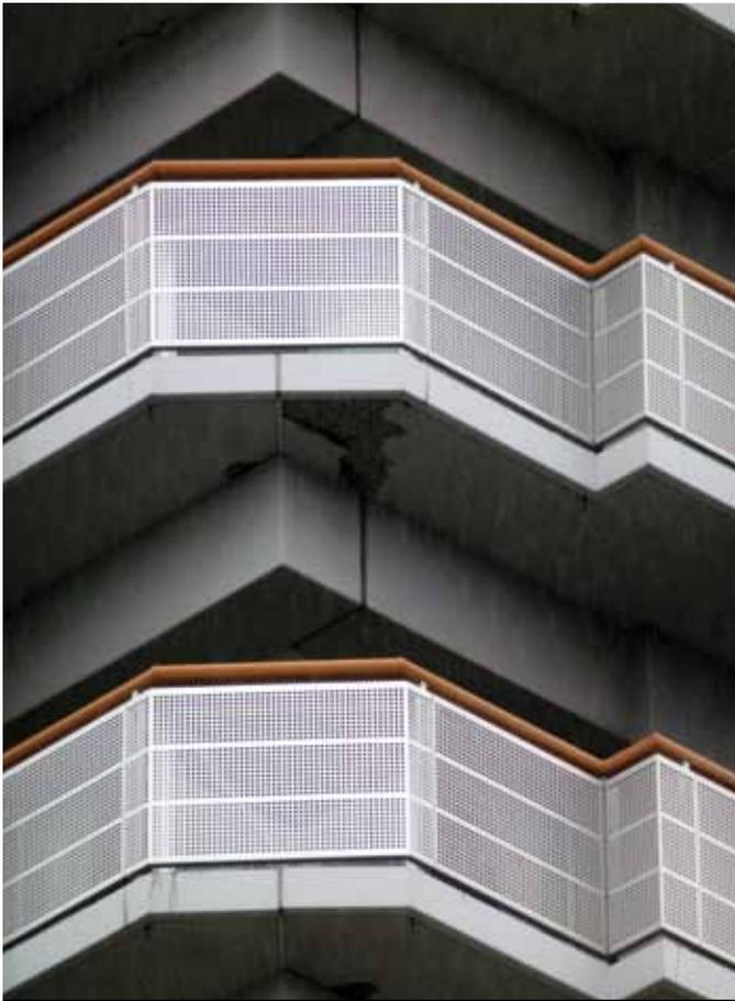
**Figure 6.** Spalling of slabs at corners of Namagachi Lions Tower.
