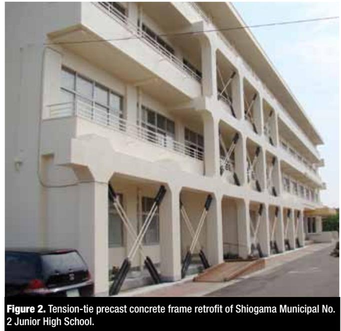
**Figure 2.** Tension-tie precast concrete frame retrofit of Shiogama Municipal No. 2 Junior High School.
