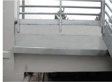
A new gutter system was installed to collect the sheet flow of rain and snow melt from the stair landing above.
