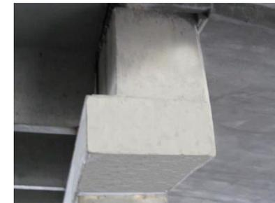
An inverted team beam and the cast-in-place ramp interface were skim coated and patched.
