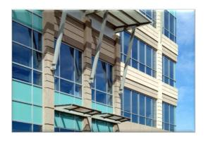
There are sections of the project where the perimiter prestressed/precast support structure has been recessed to allow the use of a unique light blue spandrel panel. This detail is repeated on multiple elevations, and on multiple levels.
