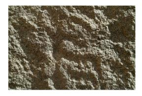
Form liner and dark tan colored acid etch precast concrete were used to mimic natural stone in the building's lower spandrel profiles.
