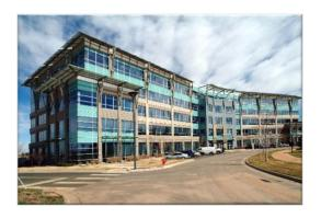
The columns are produced with the light buff color concrete and an acid etch finish, the member is exposed on all four sides, along with a four sided reveal wrap to the windows.
