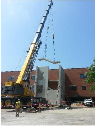
Precast stairs and landings are inserted into the shaft after the panels are erected. The exterior cores attach to the existing high school structure and allow access from the existing offices into the school.
