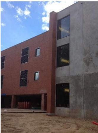
Stresscon designed the panels using a utility size brick form liner. Brick in the limited quantity and exact color replica needed for this project was difficult to find. The decision to use the form liner and then use multi-color brick stain was an effective method to accommodate the school's timeline.
