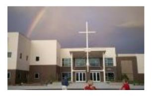
A most adaptable material, precast concrete accommodates the use of other building materials to create a cohesive appearance. At the main entrance, the brick pattern and painted surface of the panels easily incorporated the elements used for the canopy and its support structure.
