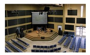
The versatile wall panels can be given a wide variety of finishes. A blue and biscuit colored paint treatment was applied to the form side of the Welcome Center's wall panels. The reveal pattern is an extension of the pattern used on many of the exterior surfaces and unifies the interior and exterior of the structure.
