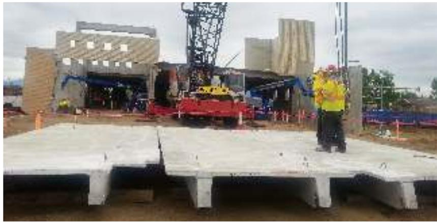
requirements and reduce required on-site installation time. All pieces were cast at Stresscon's Colorado Springs plant, shipped to the project site, and quickly erected. The significance of the hospital's mission required that new facilities be erected quickly to keep pace with the growing demand for services. The open floor design requires double tees spanning 72 to 78 feet, creating a roof system with no interior load bearing elements.
