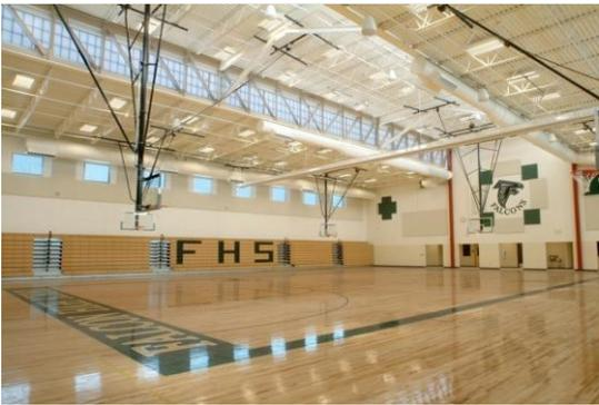
Insulated wall panels were used in the gymnasium and auditorium to reduce energy expenditure. The dual-purpose truss wall functioned as both an architectural skin and a structural load-bearing element. In addition, it provided the benefit of a high R-value. Panel interiors were given a hard trowel finish, forgoing the need for and expense of additional surface treatments.
