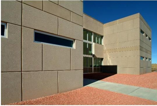
Approximately 91,000 square feet of prestressed wall panel area was erected in less than five weeks. Fabrication of the panels on a permanent long line facility allowed eight to ten panels to be cast simultaneously, resulting in decreased labor costs and an accelerated project schedule. By prestressing the panels, inherent structural advantages were realized.
