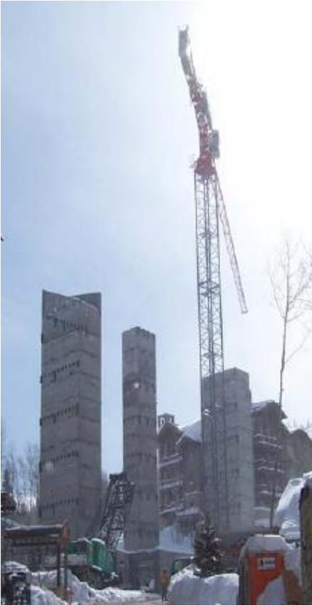
Casting enables the cores to be stacked vertically, and then the precast stairs and landings are inserted into the shaft. The integration of the elements is performed with in-house modeling to ensure the correct fit.
