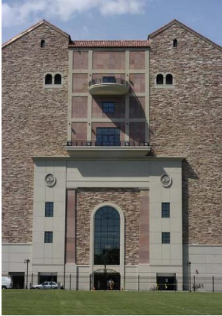
The base of the towers includes acid-etched, buff-colored concrete, and the remainder of the towers utilized the traditional local flagstone that is the prevalent architectural material employed throughout the University of Colorado campus. There are large acid-etched exterior walls with the school medallions cast on the outside entrance. The interior walls also have an acid-etched finish.
