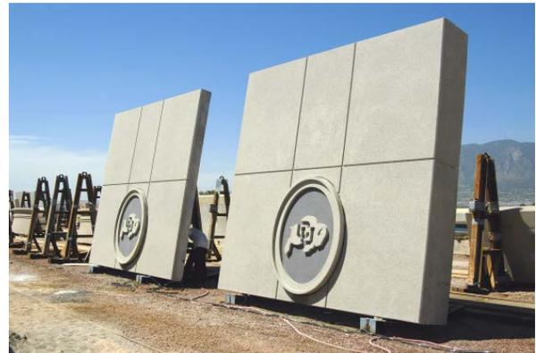
Precast concrete was erected on site at the center stair and elevator shafts. These towers create lateral stability and do an excellent job of resisting wind and earthquake loads. The individual panels are stacked on top of each other in the tower shafts using horizontal panel joints.
