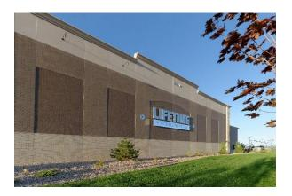
The twelve inch Thermomass wall panels were produced on a long line production facility, allowing for prestressing of the walls to maximize the structural capacity and create an economical, architectural wall panel. Thin brick was cast into the wall panels with the use of a 1/3 running bond form liner and the required architectural face mix to brick color match. The wall panels are designed to meet ASHRAE requirements, project economies, and insulation requirements.
