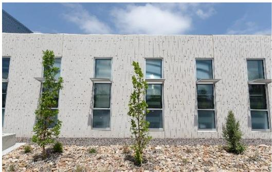
The twelve inch Thermomass wall panels were produced on a long line production facility, allowing for prestressing of the walls to maximize the structural capacity and create an economical, architectural wall panel. The wall panels are designed to achieve a steady state R-value, meeting project economies and insulation requirements.
