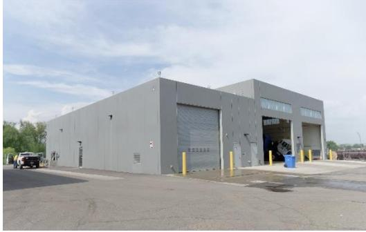
The precast panels feature an architectural gray and white acid-etch design with multiple colors and simple detailing to blend the new buildings with existing campus color schemes. With edge to edge insulation, the wall panels achieve an R-value well in excess of the ASHRAE 90.1 requirements for all wall systems.
