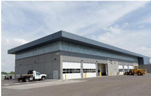
High-performance insulated precast concrete wall panels were chosen to add durability and energy efficiency to the project, and to meet specific city requirements. Loveland Service Center is the City's second LEED certified building project, recognizing building strategies and practices for high-performance green buildings. Use of local materials in the precast concrete panels contributed to LEED points.
