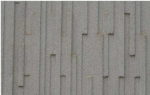
Using various precast panel types and an original form liner design allowed for aesthetic architectural detailing on the facade of the building. The custom form liner sections removed the need for an extensive and time-consuming detailing process, and created design appeal and a visually aesthetic view of the building façade.
