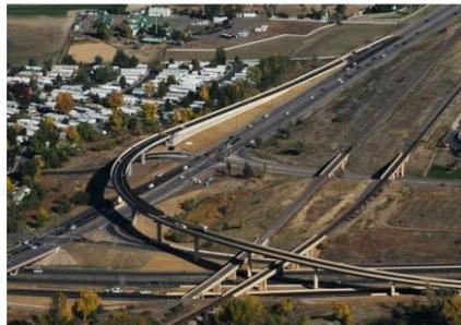
Precast prestressed girders pass above the existing railroad bridges during installation. The tub sections are installed on temporary shoring towers and post-tensioned together. Once the bridge deck is complete the shoring towers are removed.
