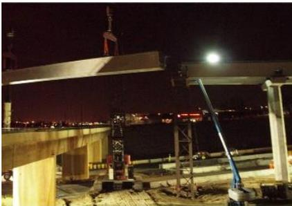
The curved precast girder is being set on falsework at one end, and on a precast pier cap at the other. Erection is completed at night to minimize disruption to the travelling public.
