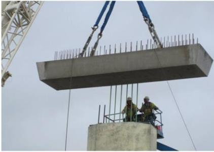
Precast prestressed pier caps are threaded over bars projecting from the pier caps. Note the use of turnbuckles to ensure the pier cap hangs in the correct super elevated position. Despite the piers being cast on site and the pier caps being plant cast, the fit is perfect.
