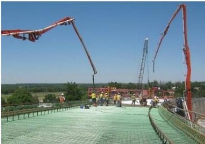
A cast in place deck placement shows two pump trucks and a finishing machine working on the bridge section.
