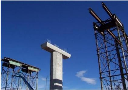
The curved tub sections are installed and supported at each of these complete pier cap and temporary shoring towers as shown in the image. Temporary shore towers are used to support the simple span while infill pours of post tension are installed.
