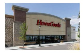
Big box characteristics, such as a rectangular shape, flat roof and ceiling trusses, and concrete walls clad in masonry, are also reminiscent of Victorian period construction. While the shops retain many big box qualities, a higher level of architectural treatment was applied to their design. The store's entryway spandrel is curved and flanked by multiple-height columns, incorporating arches and strong vertical lines distinctive of the period.
