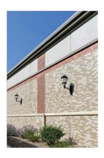
Ten different colors of brick created five blends that composed the architectural skin of the shops. One phase utilized form liner to mold a brick pattern in the wall panels at the rear of the stores. The pattern was then painted to give the appearance of real brick, resulting in significant cost savings. Of the project's 61,320 square feet of exterior wall area, 22% consisted of inset thin brick and 12% consisted of a brick pattern shaped by form liner.
