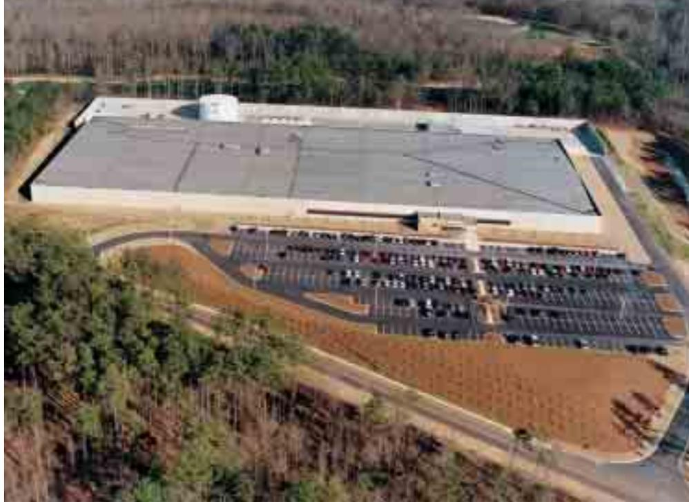
*The all-precast structure was designed to withstand 200-mph winds. The 995 precast components were erected in only five weeks, bringing the 254,000-square-foot facility on line in record time.
