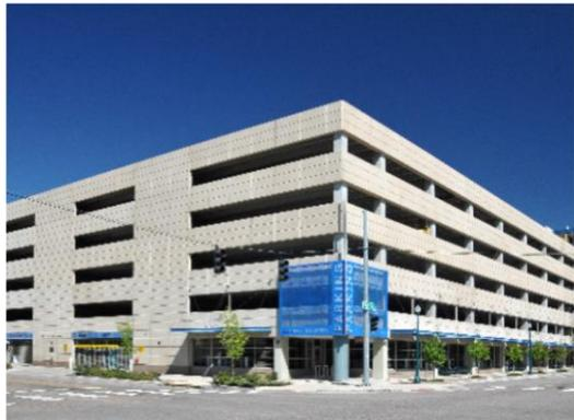
To reduce the scale of the structure without sacrificing space, horizontal precast wall panels were incorporated into the design. The combination of uninterrupted bands of panels and long openings for natural ventilation furthered the impression of a lower, wider silhouette. Exit and entrance ramps were placed at the rear corner of the structure, allowing the storefront to face pedestrian-heavy Tejon and Costilla for a more pleasant view.
