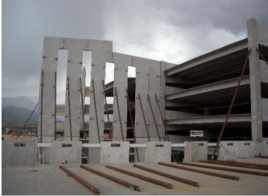
Extensive shoring was required for the interior light walls as they stacked an additional forty feet on top of the existing light walls. The new levels contributed an extra 140,500 square feet to the former 111,000 square foot parking structure. 439 supplementary parking spaces were created, raising the total number to 788.
