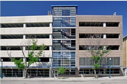
Great care and attention to detail was paid to enhance the appearance from Tejon Street. The complementary-toned panel and spandrel systems on either side of the glazed stair tower provide visual interest and appeal, and the consistent use of blue for the canopies and top of the tower unifies the structure horizontally and vertically.
