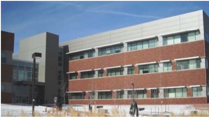
Brigade and Battalion Headquarters, Fort Carson, CO LEED Gold Certified
