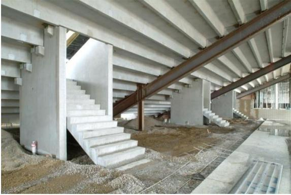
The precast/prestressed concrete used in the structure consists of 581 pieces. These include 441 pieces of single leg risers, five pieces of triple risers, 117 pieces of walls and beams, and 18 stairs.
