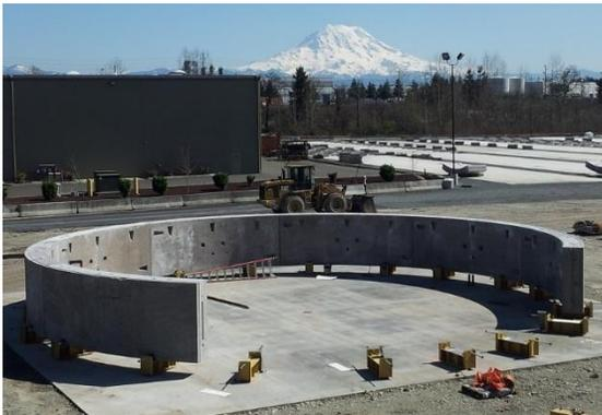
Tunnel segments will be placed to a maximum depth of 200 feet below sea level with a maximum pressure of 5.6 bar. The segments are produced to provide 100 year service life. The precast pieces are also rated for a magnitude 10 earthquake.
