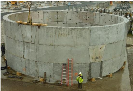
The SR99 Tunnel is composed of 10 segments per ring. The ring contains seven A segments, two counter key segments, and one key segment. Each ring has a two foot thickness. They have an internal diameter of 52 feet and a width of approximately a 6'-6". The average segment weight is 38,000 pounds. The tunnel length is 1.8 miles and will include a total quantity of 1,445, or 14,450 segments.
