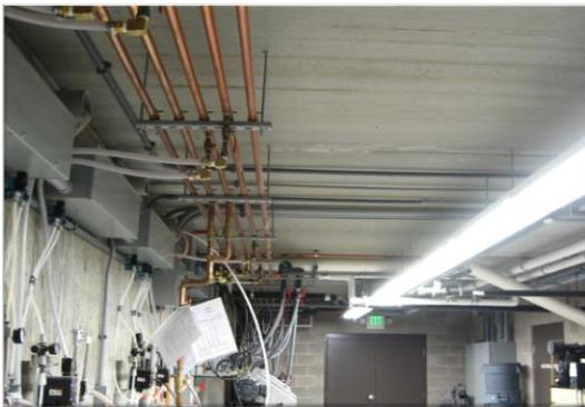
The space below the floor housed the mechanical equipment and required multiple penetrations. A hollow-core system offers this type of flexibility, and these penetrations are easily installed on site with minor adjustments for reinforcement.
